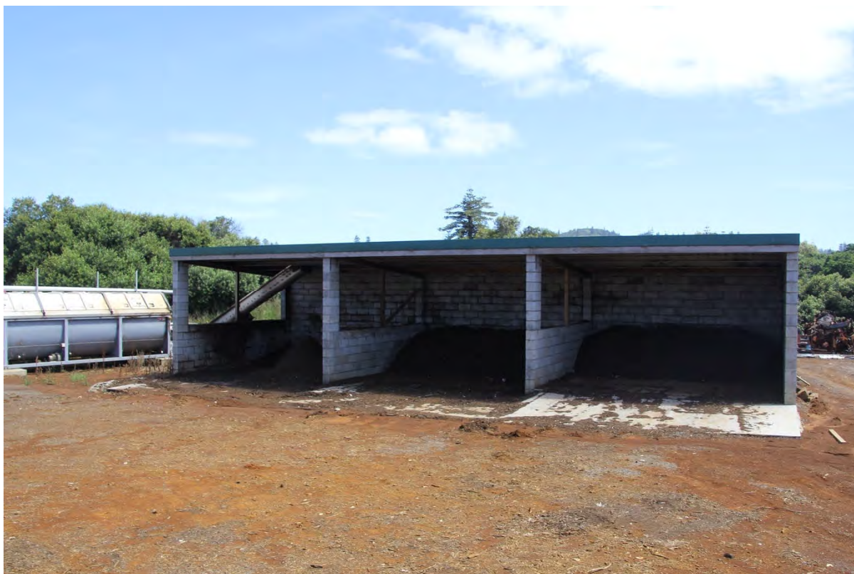
Figure 3.16: Hotrot Compost receival bays
