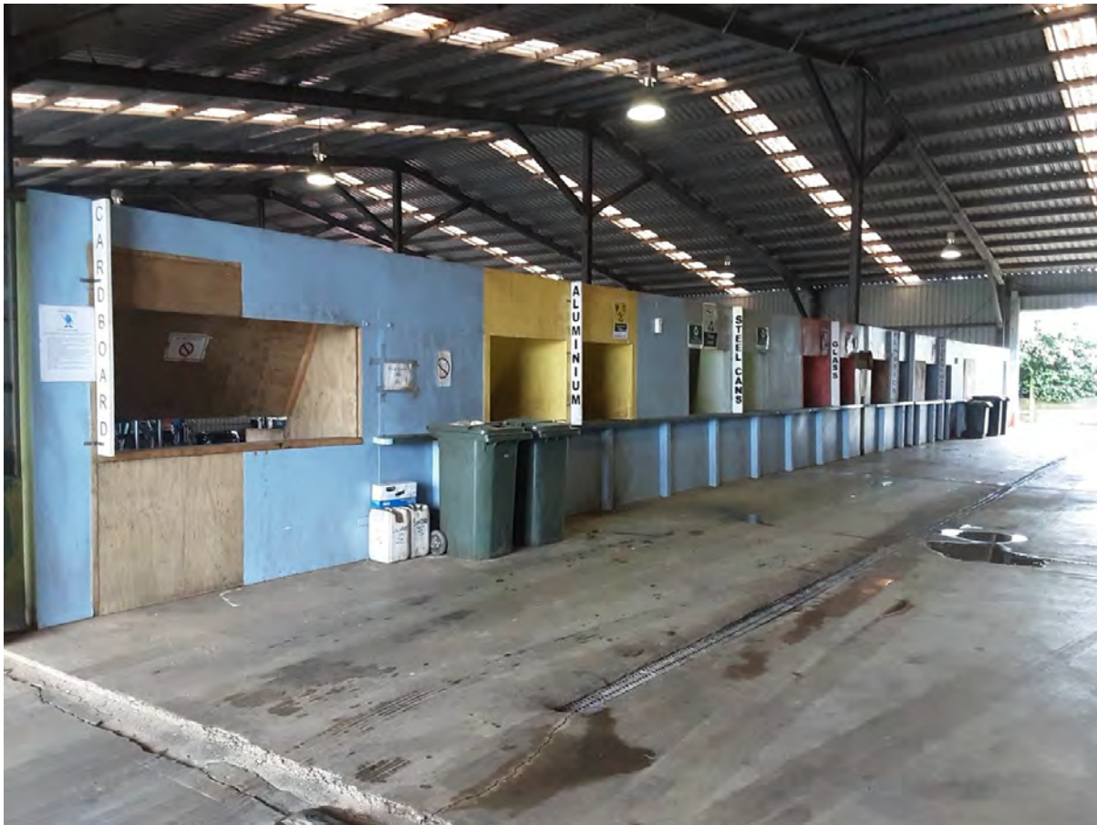
Figure 3.2: Norfolk Island WMC waste drop off area and disposal chutes 2020
